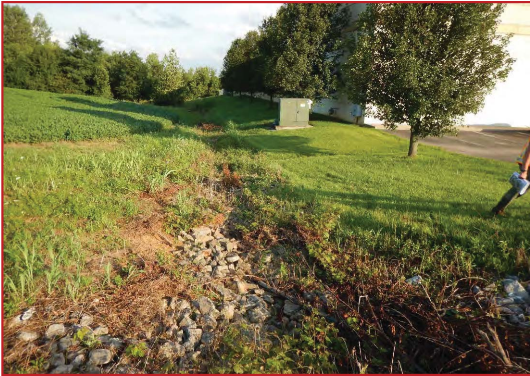
Photo 39. Looking northwest along riprapped ditch, north of New Middle Road
